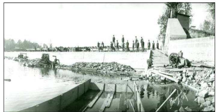
Bronson photo showing the building of the dam at Independence. It was built to provide water for the canal system. The wooden dam was replaced in 1924 by concrete.
