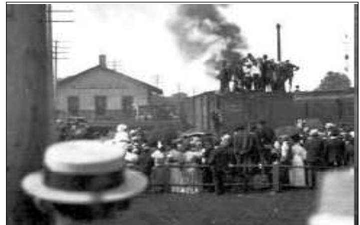
Built in 1875, this union station was on the east side of Deatrick Street SE of Harrison Avenue. Although built by the B&O, the station had platforms on both sides to serve both the B&O and Wabash.
